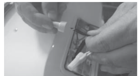
Figure 18 - Connecting the electrical wires.
